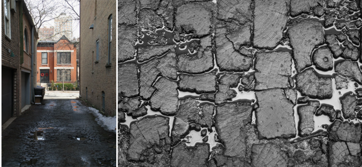
Above: Another example is in Lincoln Park; there is a small east-west alley south of Webster and west of Hudson. It is in incredible disrepair, a good illustration of Nicolson pavement's great shortcoming.
